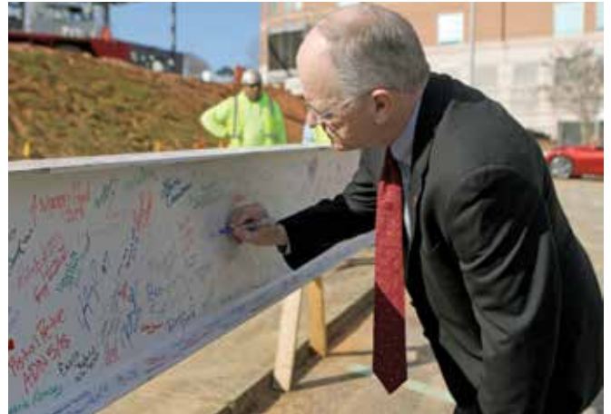
Dr. Booth signs the beam before the last piece of structural steel is placed.
