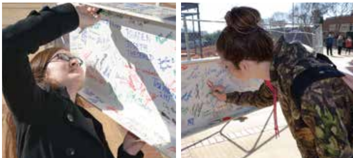
For several days prior to the topping off ceremony, students flocked to a tent set up on Fulp Plaza to sign the commemorative steel beam.
