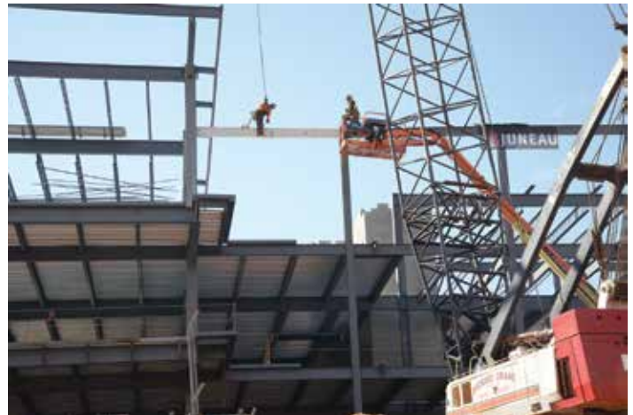
Juneau Construction workers placed the last steel beam as part of the topping off ceremony for the Student Success Center.
